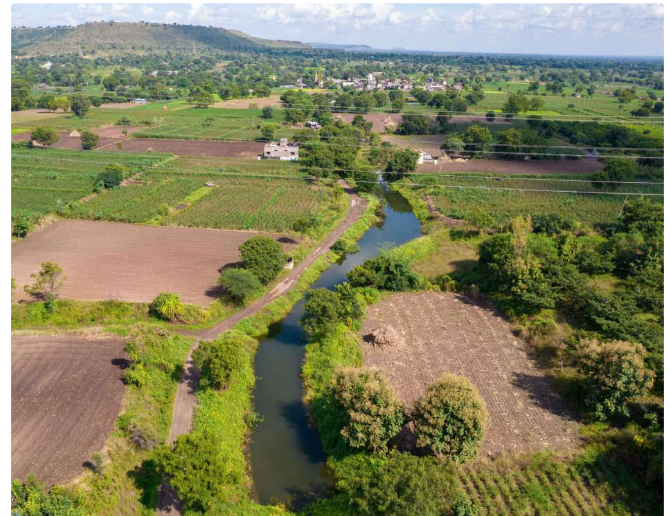
Canal deepened to increase water capacity
